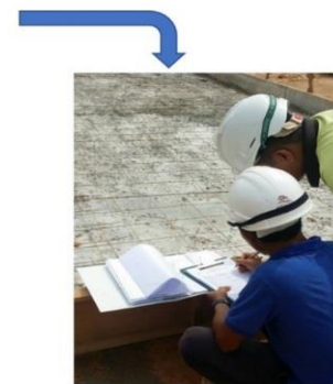
Inspection of Work
