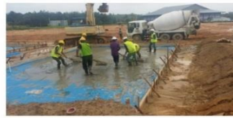
Preparation of Lean Concrete
