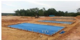
Preparation of Formwork
